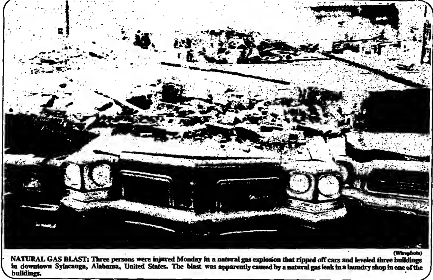
NATURAL GAS BLAST: Three persons were injured Monday in a natural gas explosion that ripped off cars and leveled three buildings in downtown Sylacauga, Alabama, United States. The blast was apparently caused by a natural gas leak in a laundry shop in one of the buildings.
